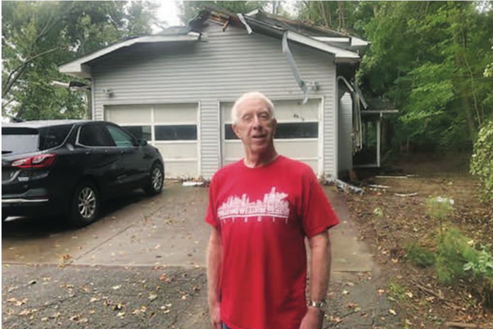
Ronald Hartley, who lives in Conway Township with his wife, stands in front of the garage that was damaged by the storm that hit the area on August 24th. With 21 trees located on his property that were either uprooted or had their tops snapped off, he believes a low-level tornado caused the damage, not just a very strong wind.
