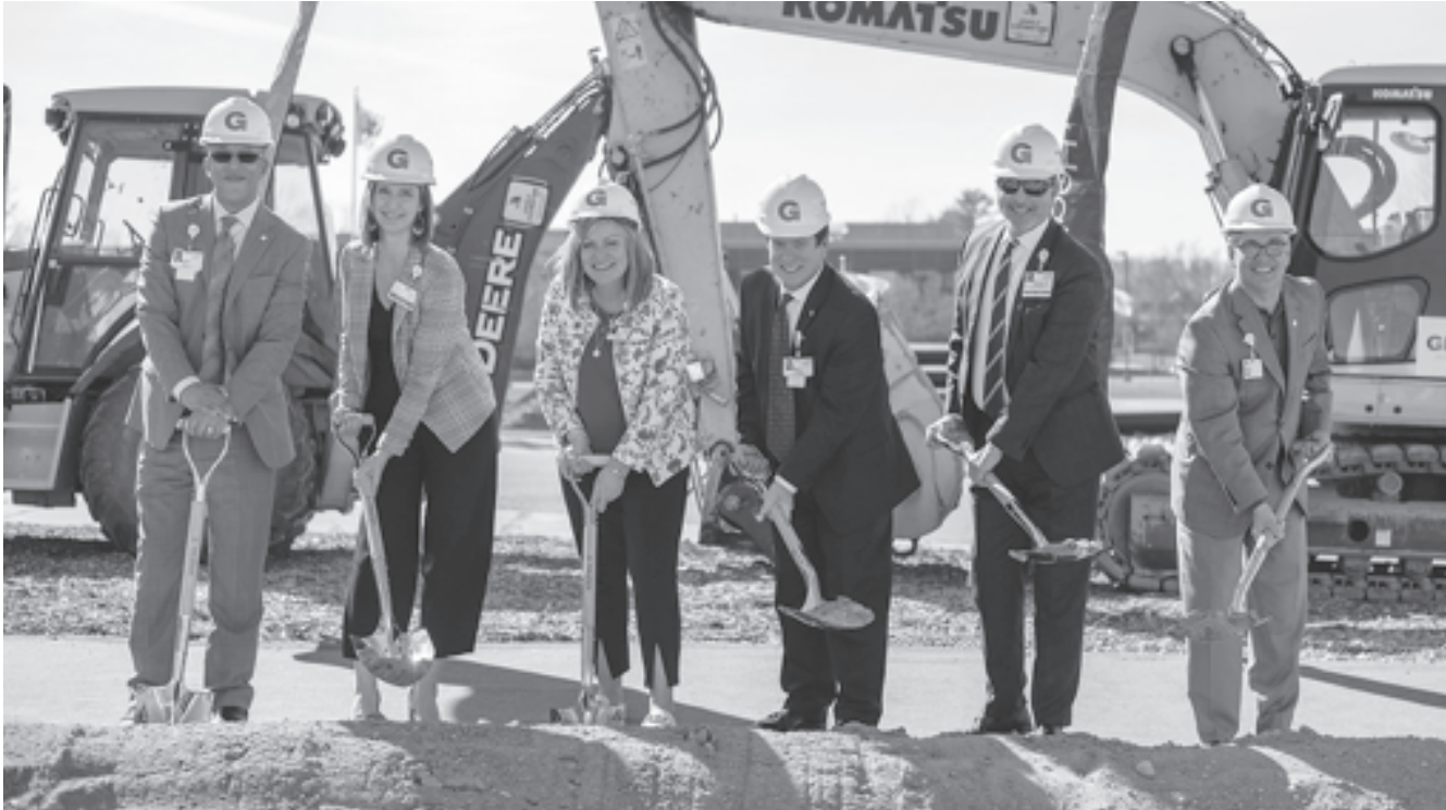
Local caregivers and executives from Trinity Health Michigan came together on Thursday, April 13 to celebrate the groundbreaking of the new Trinity Health Livingston hospital.
