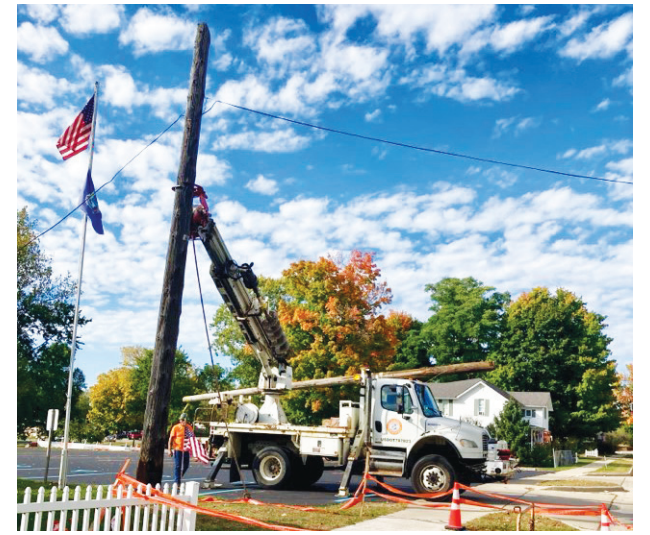
AT&T removed a telephone pole that had decayed.
