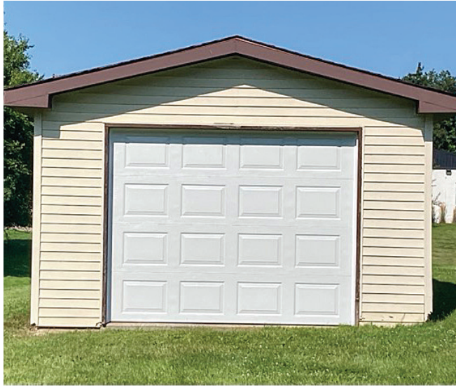
A new door was installed on the Storage Building.
